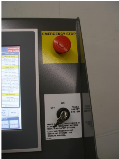
Emergency Stop Button & Keyed Safety Reset Switch
