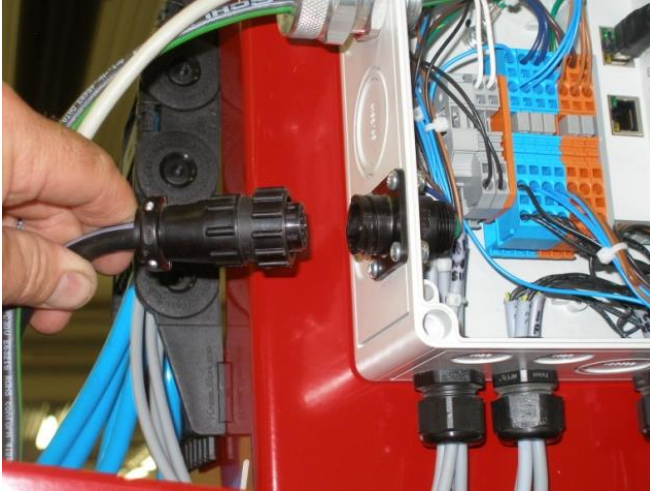
Plugging in the Electrical Connection
