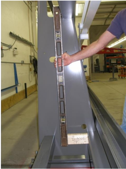
Plumbing the Guide Tubes
