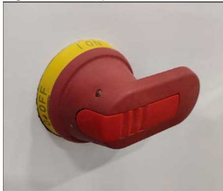
Figure 1-1: Sample of a Disconnect Switch in Off Position
