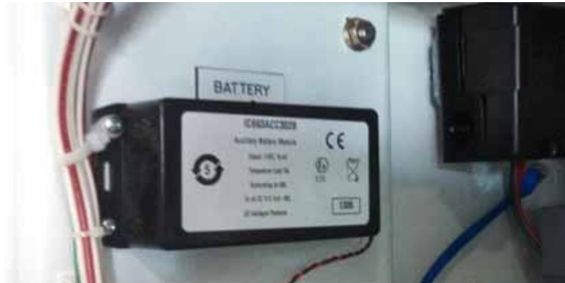
Figure 9: Remove the Old Battery Module
