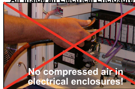
Figure 7-1: Never Use Compressed Air Inside an Electrical Enclosure
