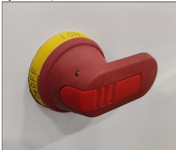
Figure 1: Example of a Disconnect Switch in the Off Position
