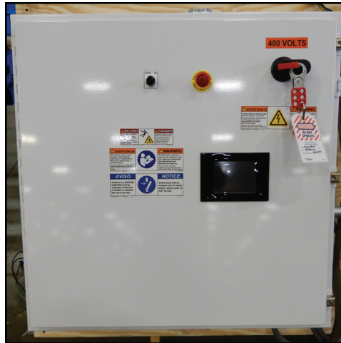
Figure 2: Sample of a Lockout/Tagout Mechanism on an Electrical Enclosure
