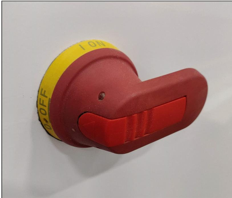
17. Turn the disconnection switch to the on position to restore power.
